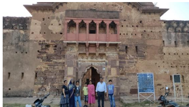
Fig. 7. Dilapidated Keoti Fort constructed taking advantage of natural obstacles for safety. Note use of local geological rocks for construction of fort.
